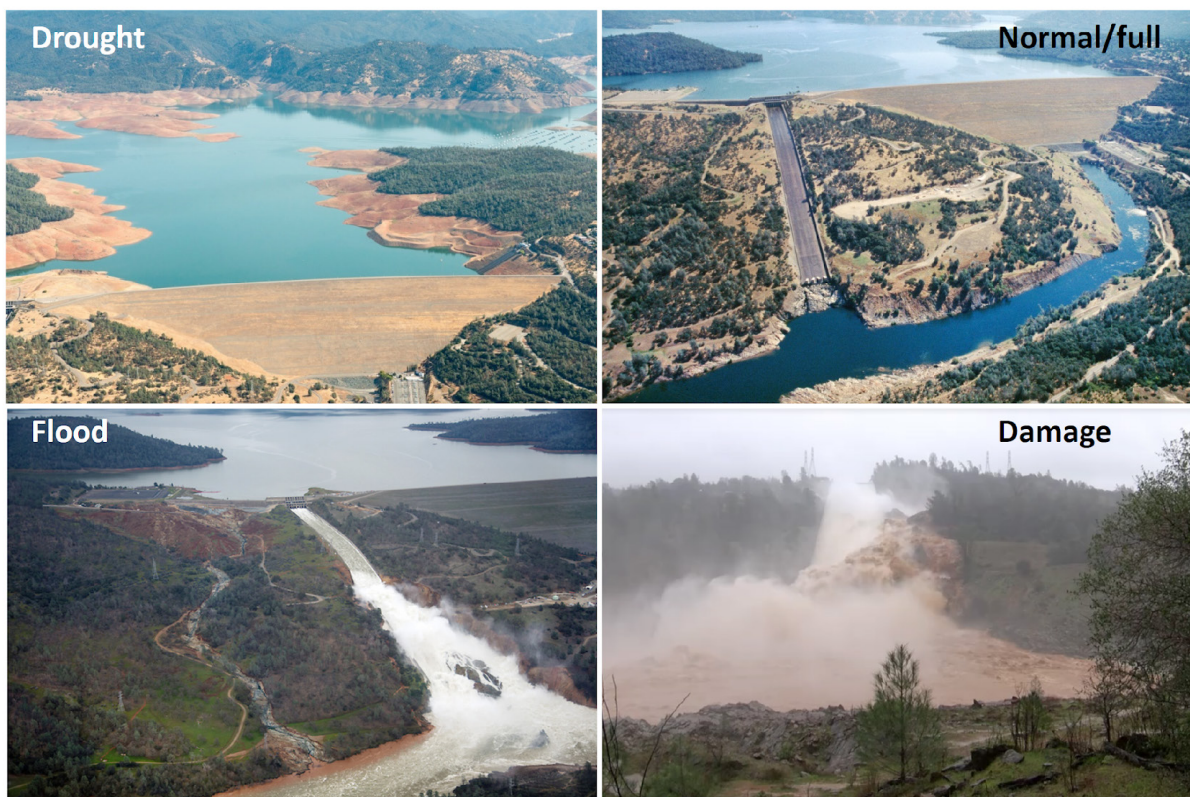
Photos illustrating the wide range of water levels at Oroville Dam and associated challenges faced in managing water in an environment of extremes, for which variability is driven by atmospheric rivers.
