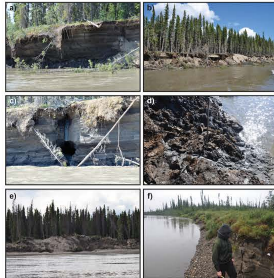
Figure 1: Images of riverbanks eroding permafrost. a) Thermal-erosion niche undercutting a bank composed of frozen sand along the Yukon River, in central AK. b) Massive failure blocks resulting from thermal erosion undercutting of banks along the Yukon River, AK (66.33° N, 147.60° W). The top of the bank is approximately 4 m above the waterline. c) Exposed ice wedge and associated bank erosion in the banks of the Yukon River, AK. d) Thermal denudation and collapse of an ice-rich bank along the Koyukuk River (65.780° N, 156.437° W). Shovel handle in center of photo for scale. e) Sediments piled up on riverbank due to river ice erosion and sediment transport on the Yukon River, AK. f) Riverbank along the Selawik River in July 2012 showing loose thawed gravels and tundra blocks from spring bank erosion protecting the bank face (66.48° N, 157.71° W).
